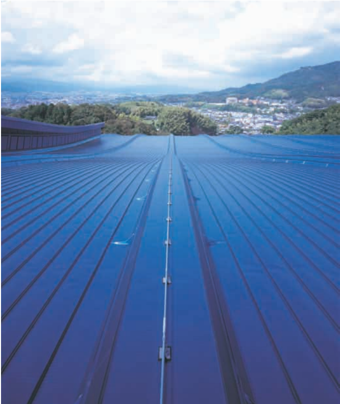
Application of edge waves ⇒ Rolling (with ribs) ⇒ Seam welding
