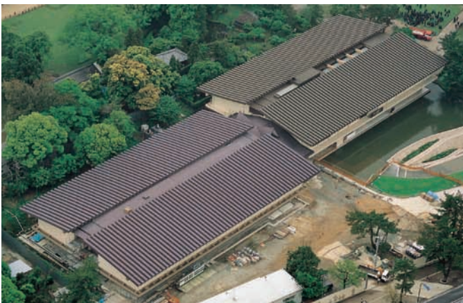
Nara National Museum (No. 2 Annex) Surface: Alumina blasting (AD03), brown coloring Area: 6,000 m 2 Weight: 12 tons Completed: 1998
