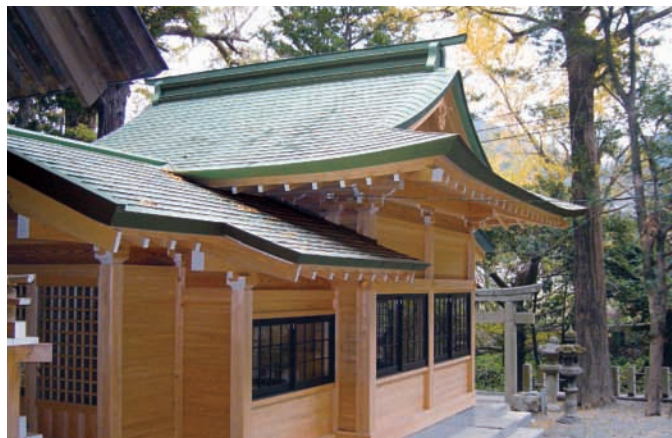
Ashitaka Shrine Surface: Alumina blasting (AD09), verdigris coloring Area: 440 m 2 Weight: 0.4 tons Completed: 2006
